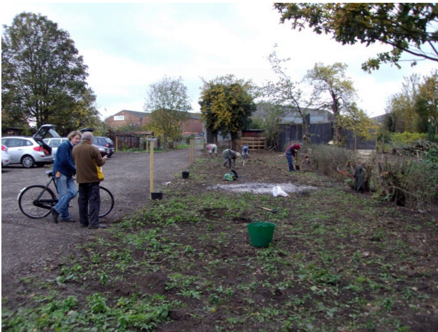
SCOG team clearing the site
